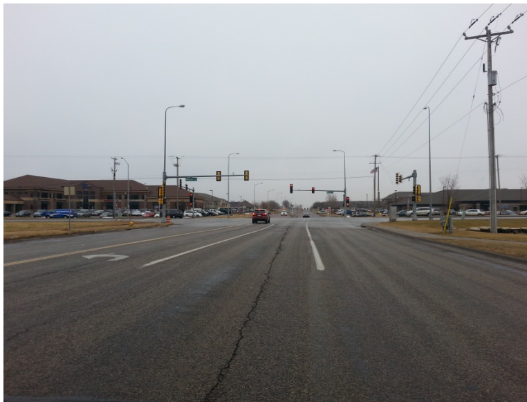
16 17 FIGURE 4 Solid Lines on an Intersection Approach
